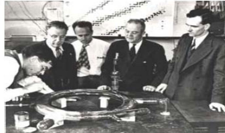
General Electric betatron built in 1946, the origin of the discovery of Synchrotron radiation.
